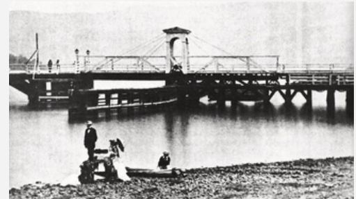
below: view of the rolling truss bridge from downstream showing tower and timber towpath for vessels. The iron wheels are visible on the right side of the tower. image via Tasmanian Heritage & Archive Office
