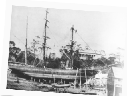
The barque Eucalyptus on the slip at Secheron, 1862 Photo courtesy TAHO
