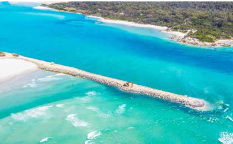
Seawall on the barway
