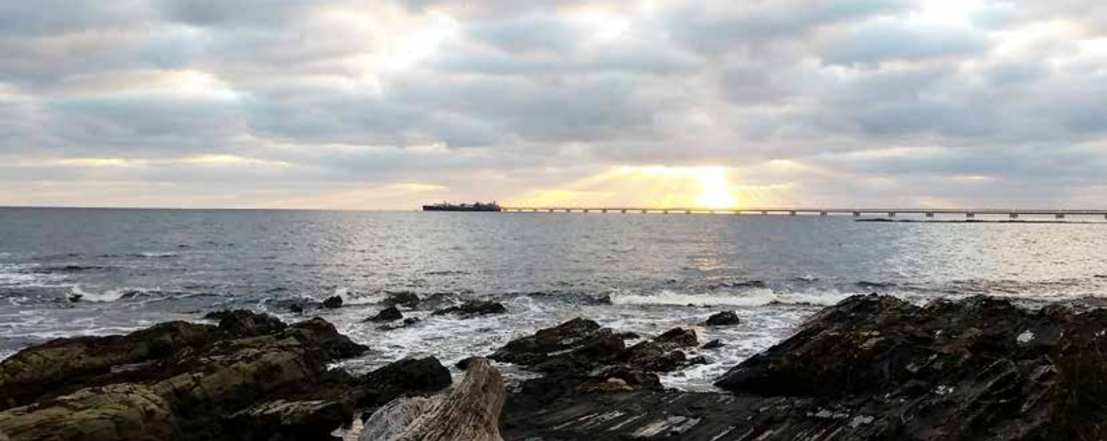
The long conveyor belt at Port Latta
