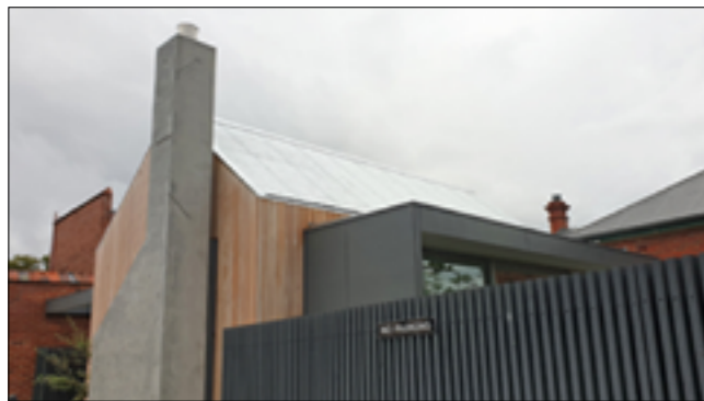
Indentations on the new chimney attached to the restored former Signalman's Quarters are imprints of telegraphic signals, which serve as a reminder of its history. Photo (2021): Rex Cox
