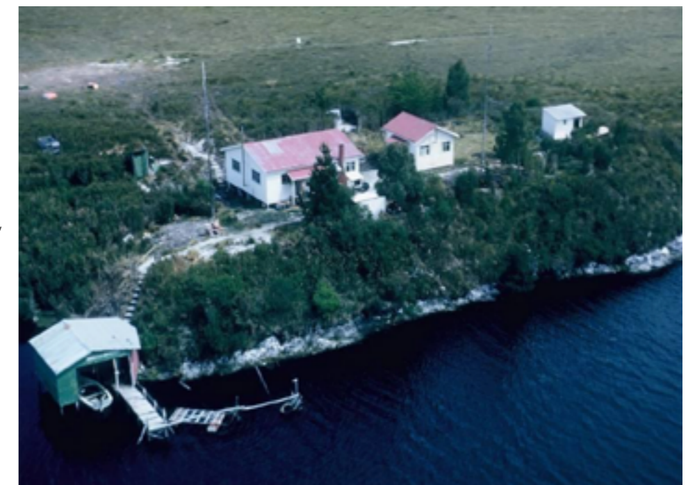
The Mines Department field station, Melaleuca Inlet, 1965, at that time occupied by BHP geologists. Photo: Mike Hall
