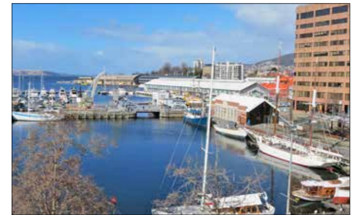
The bascule bridge which replaced the swing-bridge. It allows access by pedestrians and vehicles, and lifts to permit boats passage into and from Constitution Dock. Also visible is the steam crane. Westward is in the foreground. Photo: 2019 John Wadsley
