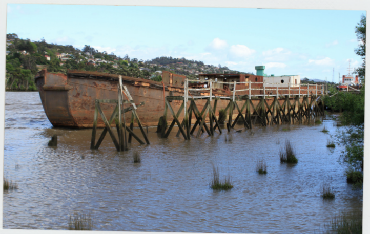
PONRABBEL II laying near King's Wharf, Launceston, 2014 (photo: Rex Cox)
