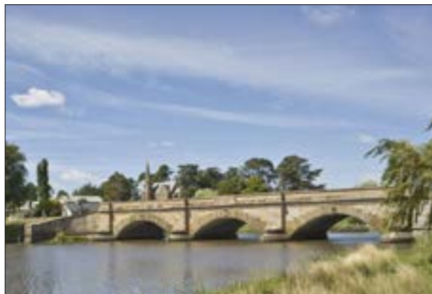
The Ross Bridge at Ross, Tasmania, completed 1836 Photo: iStock, John H
