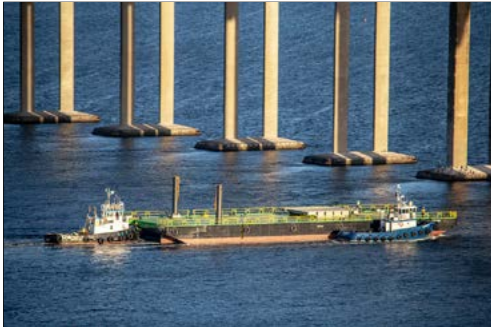
Transiting under the Tasman Bridge NBB Trust is taken to the construction site by tugs Taralga and Wandana
